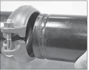
5. ASSEMBLE JOINT: Assemble the joint by inserting the grooved end of a pipe/mating component into each opening of the coupling. The ends of the grooved pipe/mating components must be inserted into the coupling until contact with the center leg of the gasket occurs. A visual check is required to ensure the coupling keys align with the grooves in the pipe/mating components. NOTE: The coupling may be rotated to ensure the gasket is seated properly.
