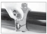
7. INSTALL BOLTS/NUTS: Install the bolts, and thread a nut finger-tight onto each bolt. NOTE: Make sure the oval neck of each bolt seats properly in the bolt hole.
