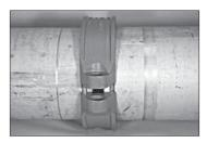
6. INSTALL HOUSINGS: Install the housings over the gasket. Make sure the housings' keys engage the groove completely in each pipe end or AGS Vic-Ring. Support the segments while preparing to install the bolts and nuts.
