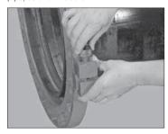
3. ADD SECOND SEGMENT: Add the second segment by inserting the draw bolts (provided) into the flange adapter with the nuts (provided) loosely and tightened uniformly. This will permit the flange adapter to be rotated for bolt hole alignment in later steps. Make sure the key of both segments engages completely in the groove.
