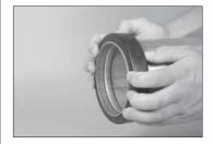
3. **POSITION GASKET:** Position the gasket over the pipe end. Make sure the gasket does not overhang the pipe end.
