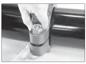
3. INSTALL BOLTS/NUTS: Install the bolts, and thread a nut finger-tight onto each bolt. For couplings supplied with stainless steel hardware, apply an antisieze compound to the bolt threads. NOTE: Make sure the oval neck of each bolt seats properly in the bolt hole.
