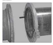
7. INSERT STANDARD, FULL-SHANK-DIAMETER ASSEMBLY BOLTS AT LAP JOINTS: Insert a standard, full-shank-diameter assembly bolt into each of the lap-joint bolt holes. Refer to the "Style W741 Helpful Information" table on the following page.
