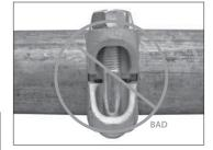
**5.** Inspect the bolt pads at each joint to ensure proper assembly is achieved.
