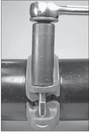
6. TIGHTEN NUTS: Tighten the nuts evenly by alternating sides until metal-to-metal contact occurs at the bolt pads. The middle section of the bolt pad mating surfaces must be in full metal-to-metal contact to ensure a properly assembled joint. Make sure the housings' keys engage the grooves completely during tightening.
