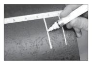
**2a.** Refer to the "Insertion Depth Requirements" table below. Using a measuring tape and a bright-colored marking pencil or paint stick, make an additional mark on the pipe ends at the measurement listed in this table. This mark will be used for visual inspection to make sure the pipe is inserted properly in the coupling. Make at least four of these marks equally-spaced around the circumference of the pipe ends.
