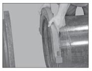
2. ADD FIRST SEGMENT: Place the first segment onto the pipe. Make sure the key engages completely in the groove. NOTE: On vertical pipe, the first segment must be held in place until the second segment is installed and fastened to the first segment. For horizontal pipe, the first segment can be balanced on top of the pipe, as shown above.
