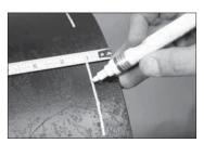
2. MARK PIPE ENDS: Using a measuring tape and a bright-colored pencil or paint stick, place a mark 1 inch/25 mm from the pipe ends. This mark will be used for reference in centering the gasket during installation. Make at least four of these marks equally-spaced around the circumference of the pipe ends.
