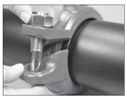
8. INSTALL REMAINING BOLT/NUT: Install the remaining bolt, and thread the nut finger-tight onto the bolt. NOTE: Make sure the oval neck of each bolt seats properly in the bolt hole.
