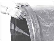
3. **POSITION GASKET:** Position the gasket over the pipe end or AGS Vic-Ring. Make sure the gasket does not overhang the pipe end or AGS Vic-Ring.
