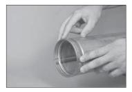
1. CHECK PIPE ENDS: The outside surface of the pipe, between the groove and the pipe end, must be smooth and free from indentations, projections (including weld seams), and roll marks to ensure a leak-tight seal. All oil, grease, loose paint, dirt, and cutting particles must be removed.
