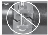
Visually inspect the bolt pads at each joint to ensure metal-to-metal contact is achieved across the entire bolt pad section.
