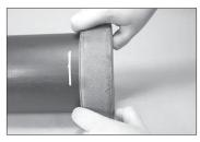
**4. INSTALL GASKET:** Install the gasket over the pipe end. Make sure the gasket does not overhang the pipe end.
