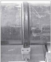
4. JOIN PIPE ENDS: Align and bring the two pipe ends together. Slide the gasket into position, and center it between the groove in each pipe end or AGS Vic-Ring.
