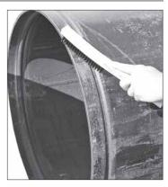
**1b.** Clean the outside surface of the pipe, from the groove to the pipe end, to remove all oil, grease, loose paint, and dirt.
