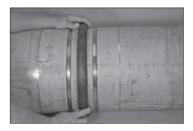
4. JOIN PIPE ENDS: Align and bring the two pipe ends together. Slide the gasket into position, and center it between the groove in each pipe end or AGS Vic-Ring.
