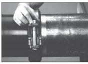
6. INSTALL BOLTS/NUTS: Install the bolts, and thread a nut finger-tight onto each bolt. NOTE: Make sure the oval neck of each bolt seats properly in the bolt hole.
