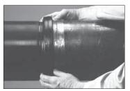
4. JOIN PIPE ENDS: Align and bring the NPS and JIS pipe ends together. Slide the gasket into position and center it between the groove in each pipe end. NOTE: Make sure no portion of the gasket extends into the groove in either pipe and that the NPS side of the gasket is facing the NPS pipe.
