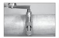
4. TIGHTEN NUTS: Tighten all nuts evenly by alternating sides. Make sure the housings' keys engage the grooves completely on both pipe ends. Apply torque to each nut with a torque wrench. Refer to the following table for the torque requirement. NOTE: It is important to tighten the nuts evenly to prevent gasket pinching.
