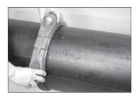
**INSTALL FIRST SEGMENT** ASSEMBLY: Install one of the preassembled halves over the gasket. Make sure the housings' keys engage the grooves completely on both pipe ends.
