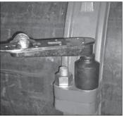
7. TIGHTEN NUTS: Tighten the nuts evenly by alternating sides (refer to the graphics in the left column of this page for the tightening sequence). Make sure the housings' keys engage the groove completely in each pipe end or AGS Vic-Ring. Continue to tighten the nuts evenly by alternating sides until metal-to-metal bolt pad contact AND the specified torque value are achieved. Refer to the "Required Assembly Torques" table on the following page.
