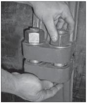
**6a. INSTALL FLAT WASHERS/NUTS:** Install a flat washer (supplied with the coupling) onto the end of each bolt, and thread a nut finger-tight onto each bolt. **NOTE:** Make sure the oval neck of each bolt seats properly in the bolt hole.
