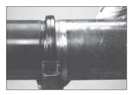
5. INSTALL HOUSINGS: Install the housings over the gasket. Make sure the larger openings of the housings (marked NPS) face the larger pipe (NPS side) and that the housings' keys engage the grooves completely on both pipe ends.
