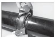
7. **INSTALL HOUSINGS:** Install the housings over the gasket. Make sure the housings' keys engage the grooves properly on both pipes/mating components.
