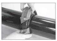
3. **INSTALL HOUSINGS:** Using the "swing-over" feature, install the housings over the gasket. Make sure the housings' keys engage the grooves completely on both pipe ends.
