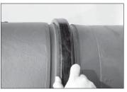
4a. If the gasket was turned inside out in step 3a for larger size (non-AGS) couplings: Roll the gasket into position and center it between the groove in each pipe end. Make sure no portion of the gasket extends into the groove in either pipe end.
