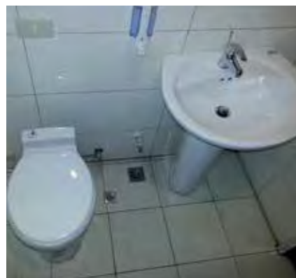
Sink connected to Sanicompact macerating toilet and pump system.
