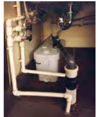
Sanivite installed underneath the counter sink
