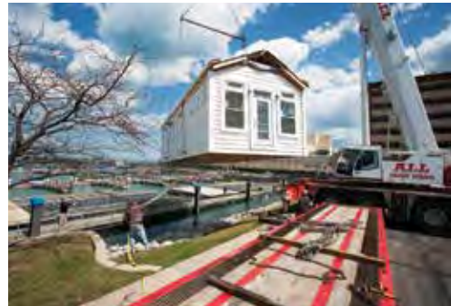
Crane used to place the bathhouse on to floats
