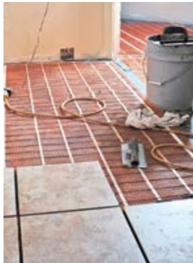
Trowel thin-set and lay tile.
