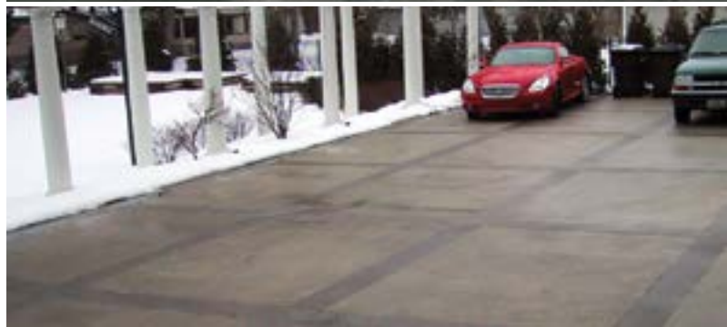
Public buildings need safe and easy access. Make plans for snow melting in walkways, stairs and wheelchair ramps.
